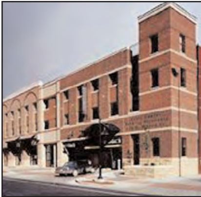
Use of historic architectural elements and materials creates a structure that enhances the Downtown Core and the pedestrian environment.
