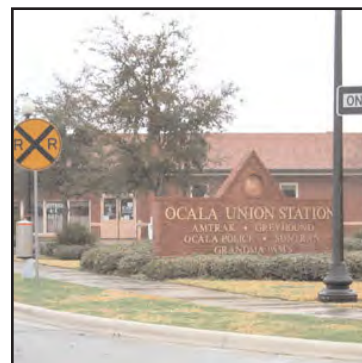
The Ocala Manufacturing site is adjacent to the Ocala Union Station, affording opportunities for future transit-oriented development.
